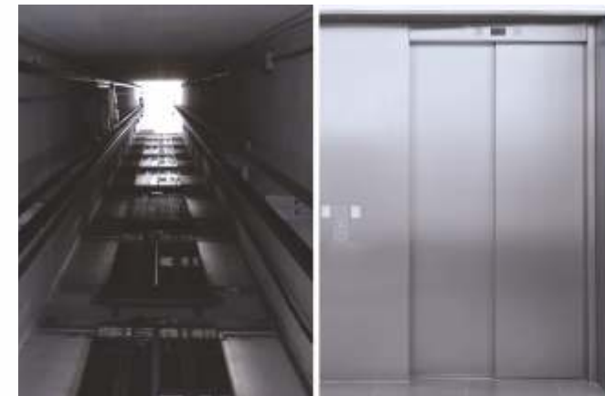
Machine room-less elevators that save on maintenance costs with 40% lower power consumption
