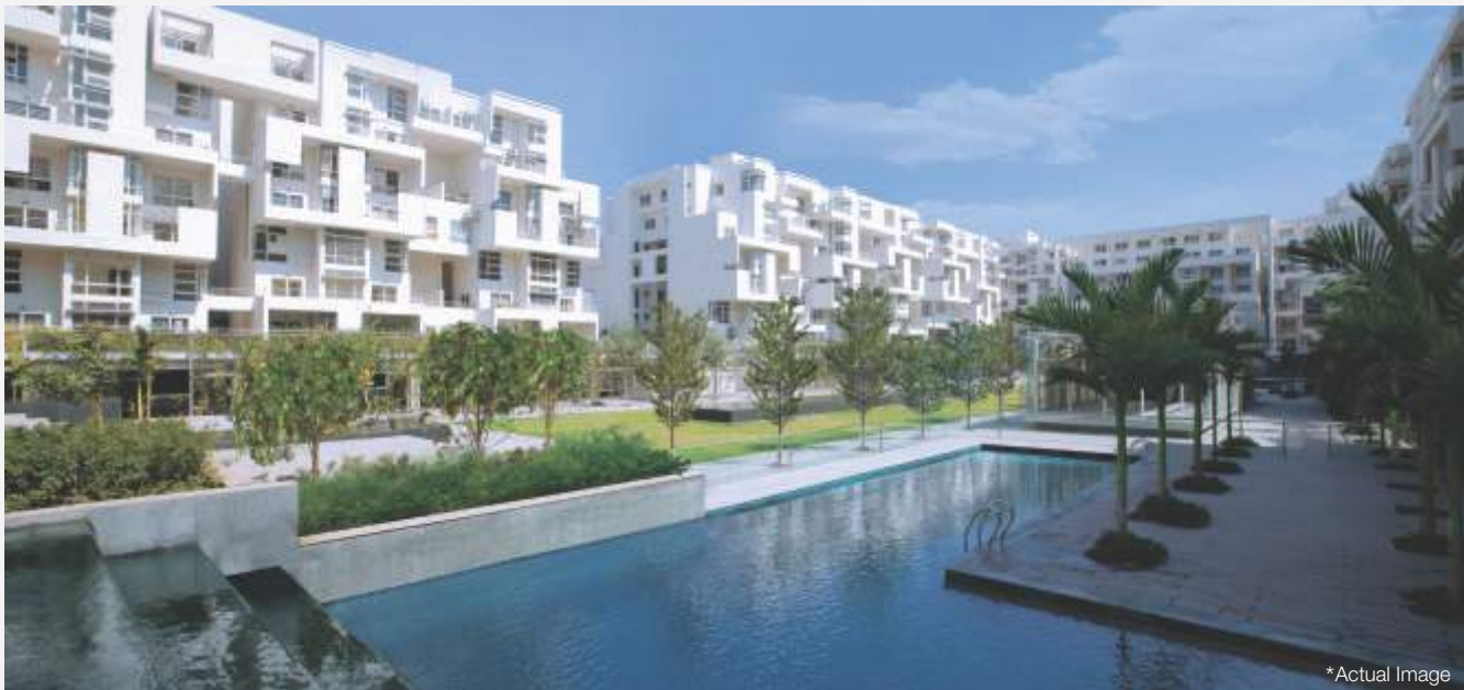
ROHAN MITHILA, PUNE Breezy, spacious homes surrounded by vast, lush-green landscape.
